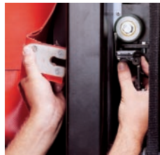
3. Reattach connecting tabs and rollers
