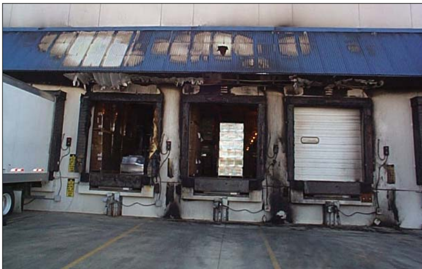
Heat-dissipating Firefighter™ headers prevent the risk of dock fires due to heat build-up from trailer marker lights.
