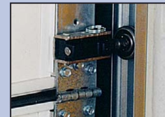
Roller assembly repositioned in track to resume operation
