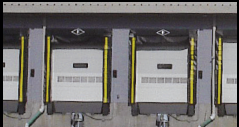
Multiple Universal GX-4000 bottom and Ventilation panels at a juice processing plant.
