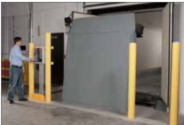
Dock attendant opens the trailer doors inside of the building and lowers the leveler into position.
