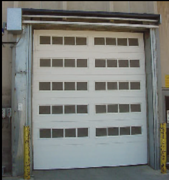
A Universal GX-4000 door with multiple Ventilation panels at a bottling plant.
