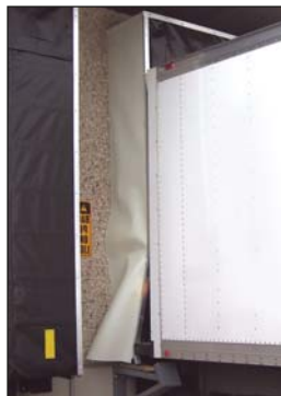
Just one trailer impact can severely damage or even destroy ordinary rigid-frame dock shelters.
