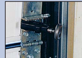
Roller assembly released following impact
