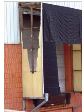
Just one trailer impact can severely damage or even destroy ordinary rigid-frame dock shelters.
