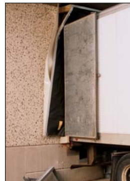
Just one trailer impact can severely damage or even destroy ordinary rigid-frame dock shelters.
